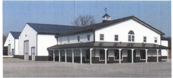
Fig. 1: Ramco Supply Facility
